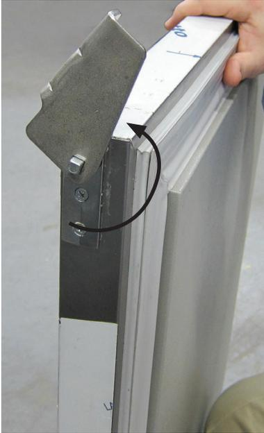
7. Hold the hinge, twist the door and slide the top pin into the top hinge.
